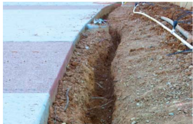
Excavating an area for sample line to monitor potential underground residual hazardous gases
